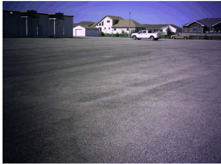
Parking lot prior to BSD
