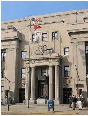
National Headquarters, Indianapolis, In
